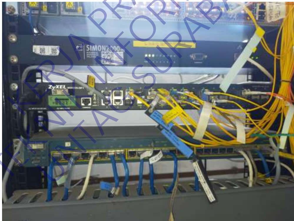
Gambar 4.13 switch zyxel
